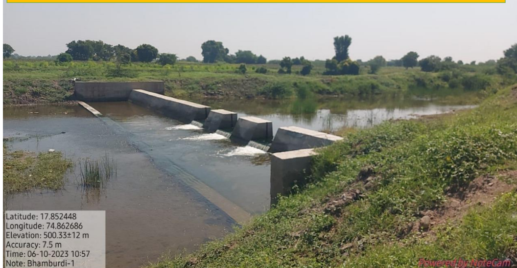
Check Dam in Solapur District, Maharashtra
